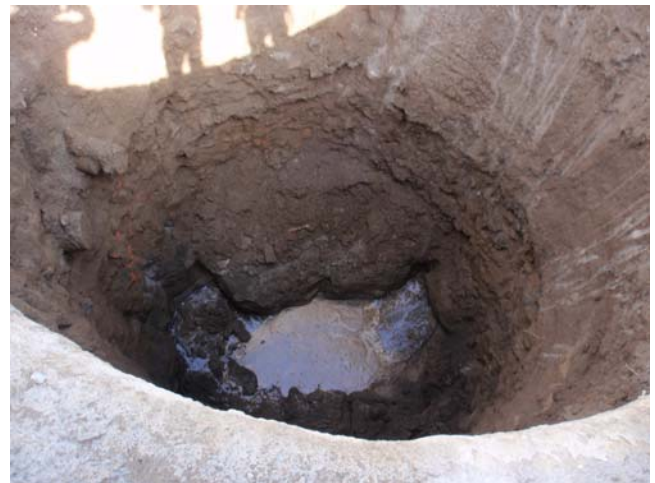
Figure 12. Missing column, left side of base
