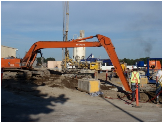
Figure 10. Excavation with long-arm backhoe
