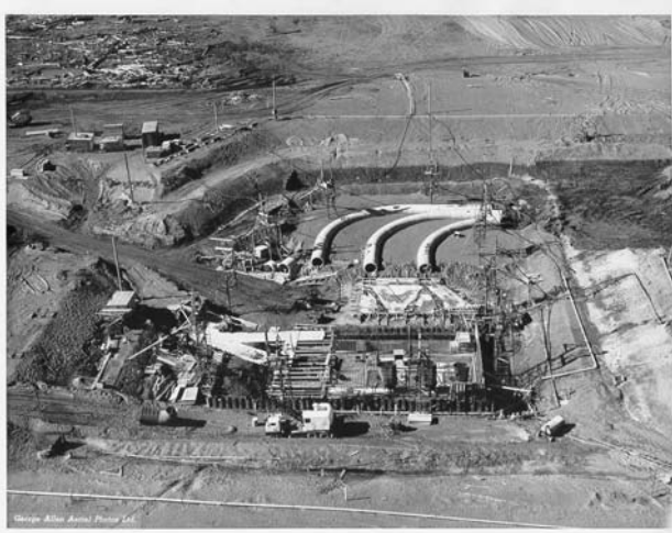
Figure 3. Aerial view of siphons during original construction
