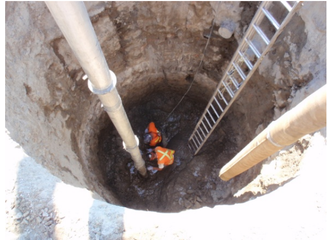
Figure 11. Completion of shaft using vacuum line
