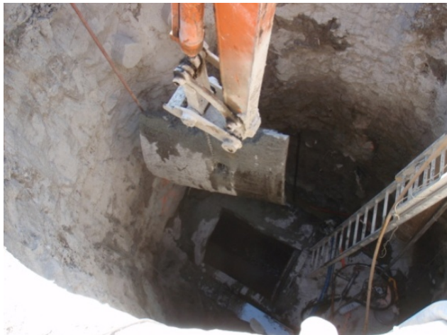
Figure 13. Completed chamber with siphon exposed
