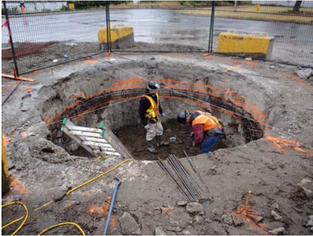
Figure 9. Shoring ring installation in upper shaft
