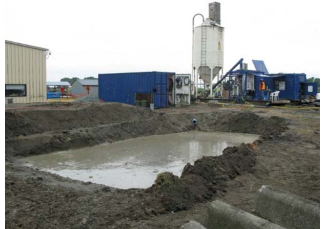
Figure 8. Mud pit and grout plant
