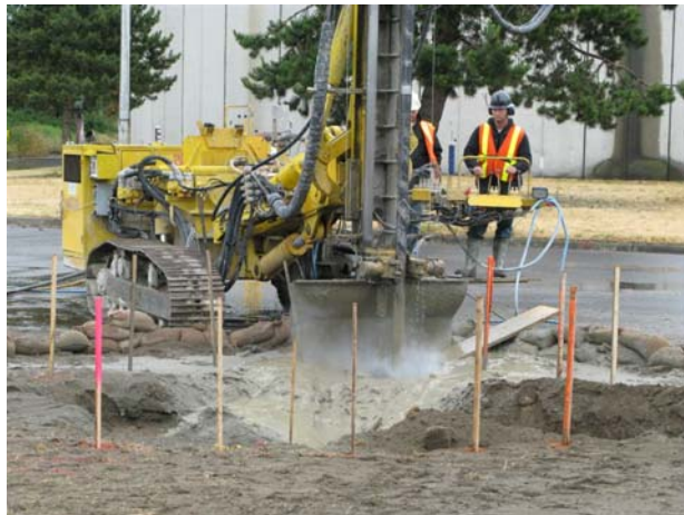
Figure 7. Drill rig excavating chamber wall column
