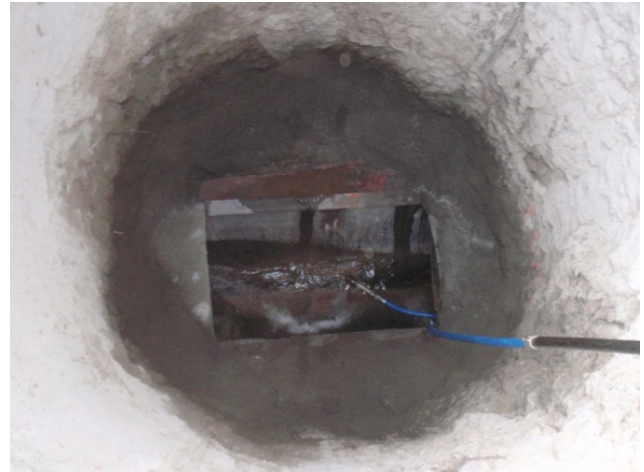
Figure 14. Final opening of the siphon
